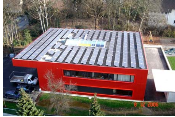
Figure 10: Ekkharthof zero-energy school building in Kreuzlingen (photo: Böhni Energie und Umwelt)
